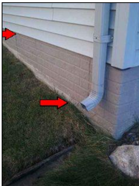
Discharge should be 6' min.
