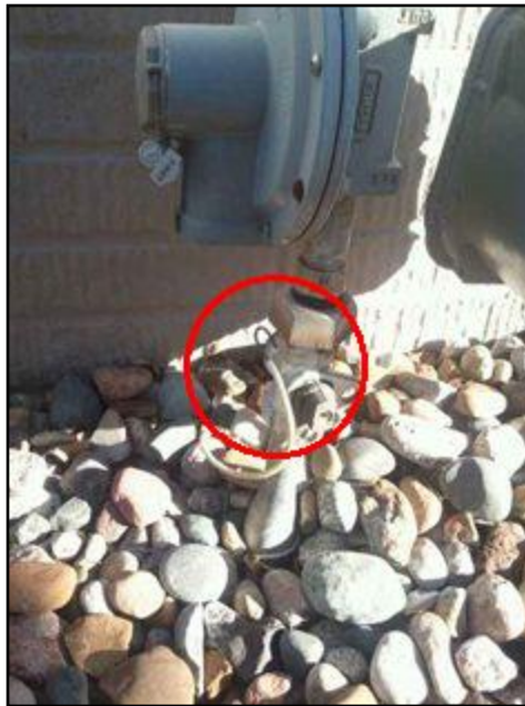
Improper connections
